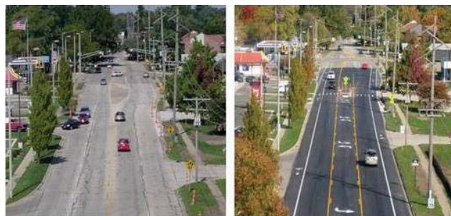
Road Diet Before (Left) and After (Right) (City of Philadelphia)
